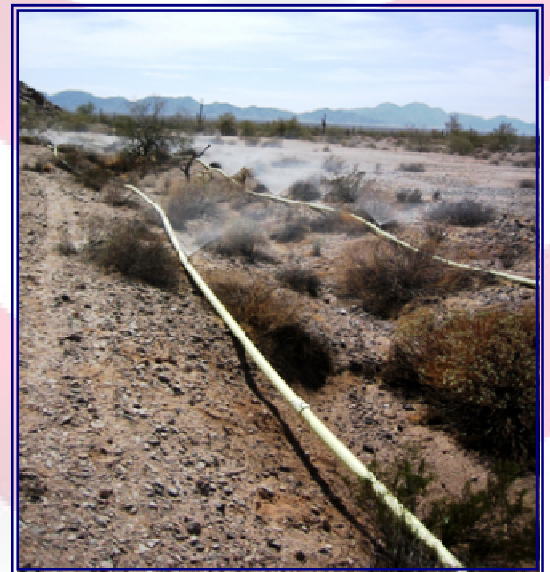
One of the new sprinkler arrays at Granite Mountains forage enhancement.
